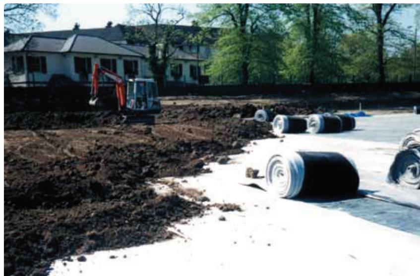
against the structure and dimpled face against the backfill, Deckdrain will also provide a high level of protection to the waterproofing system.
