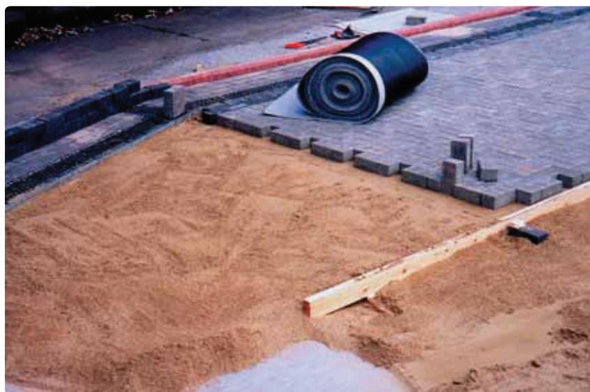
becoming saturated. Deckdrain also provides protection against puncture where a waterproofing membrane is required below the block paving (e.g. roof top car parks).
