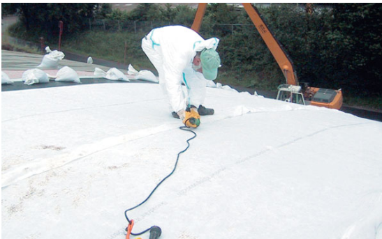
Thermal overlap fixing
