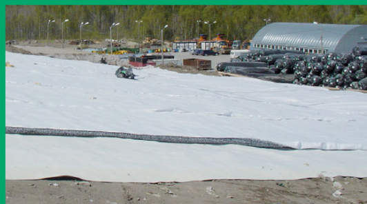
Fig. 5 Secudrain® drainage mat installed over Bentofix®
