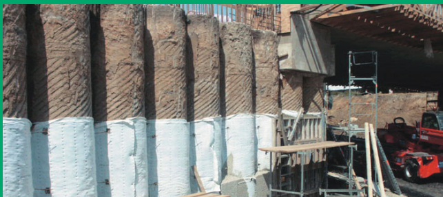
Fig. 4 Concrete was used as a level regula- ting course
