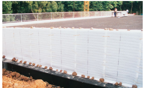
Vertical installation of Secudrain®
