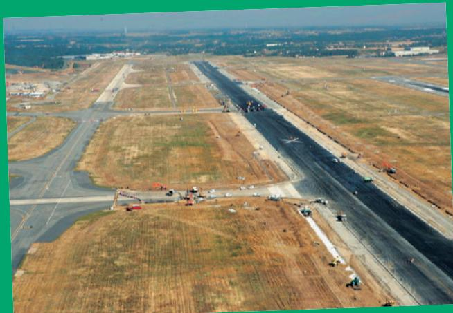
approach runways had to be completed within two months, without any hindrance to air traffic. As Bentofix® can be installed easily and extremely quickly in comparison to other conventional sealing systems, general construction work went ahead smoothly; in fact the Bentofix® installation work was completed earlier than scheduled.
