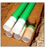
Depth of cover over conduit A minimum of 600mm depth is required from the crown of the conduit to ground level. At road crossings the minimum cover over conduit should be 800mm.
