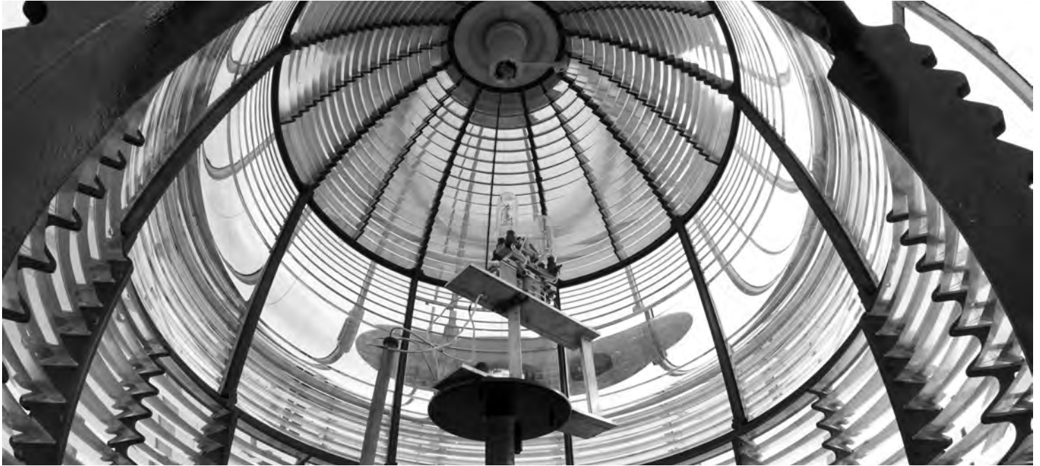
The Bodie Island restoration project cannot be considered complete until the magnificent first-order Fresnel lens is returned to the lantern room and made operational again. Lighthouse Lamp Shop, the team that disassembled the lens for safe storage during the restoration, will reassemble the lens and put it back in the lantern room during February 2013. Above is a view looking up and inside the lens canopy. Photo courtesy of De. Laddie Crisp, Jr.
