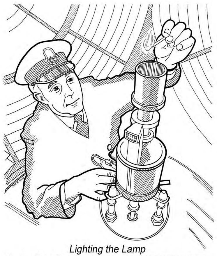
A keeper reaches up to light an incandescent oil vapor lamp, lighting the flame which will be magnified by the giant Fresnel lenses behind him to be seen by ships twenty miles out at sea. Before electric lamps and beacons, many different types of oil lamps were installed in American lighthouses to find the best and the brightest flame that would burn throughout the long nights.
