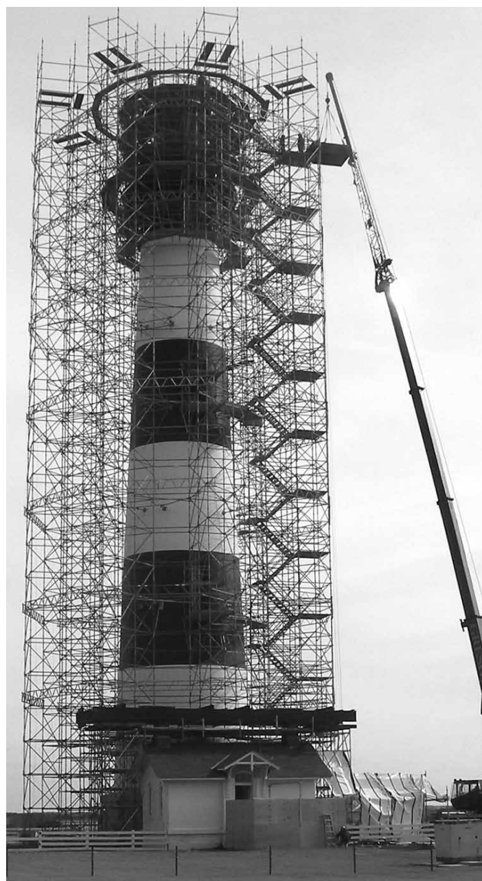
Above is the 12-story, 2,000-piece scaffolding that now surrounds the lighthouse and allows access to all exterior areas of the tower. The tall crane is one of only a few in the country that can reach 165-foot heights. The keepers' quarters and grounds remain open at Bodie Island.
