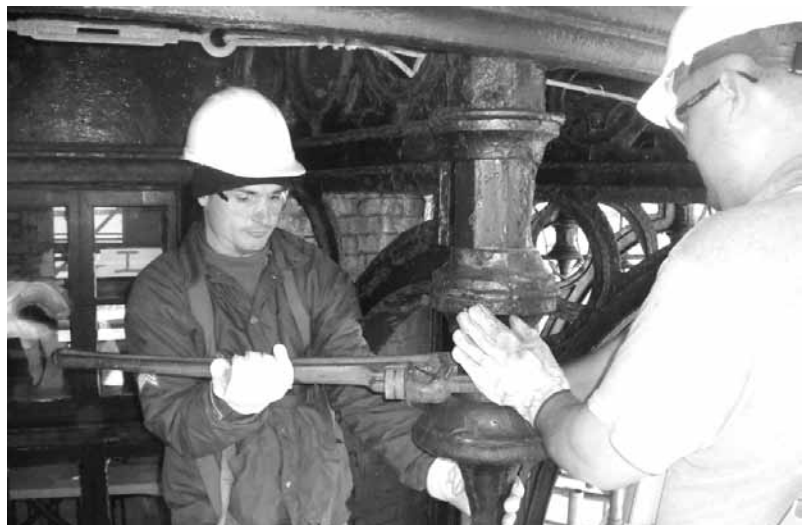
Above, workers use a gigantic wrench to persuade one of the corroded support brackets to give up its pointed "acorn." It will be removed, a wooden pattern created around which a resin-coated sand mold is made. It will be melted down at a foundry and strengthened. Corrosion, commonly known as rusting, typically produces oxides and/or salts of the original metal that build up around the iron, causing a loss of the original iron, also called "loss of historic fabric." Each acorn originally was attached by an iron rod to the top of the safety rail at the gallery deck level, but these rods have corroded to the point of being virtually nonexistent. A corroded part within another makes the work doubly difficult.
